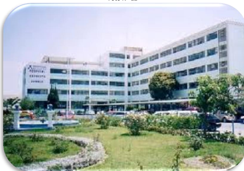
Hospital Regional Hipólito Unánue
