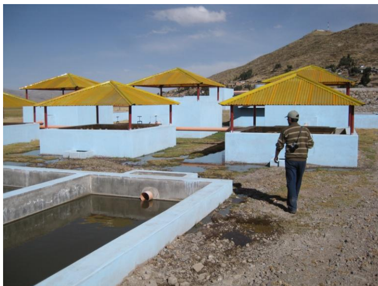
Figure 2. Leaking wastewater system pipes around the gravel filter bed treatment processes in Pomata, Peru on July 16, 2010.
