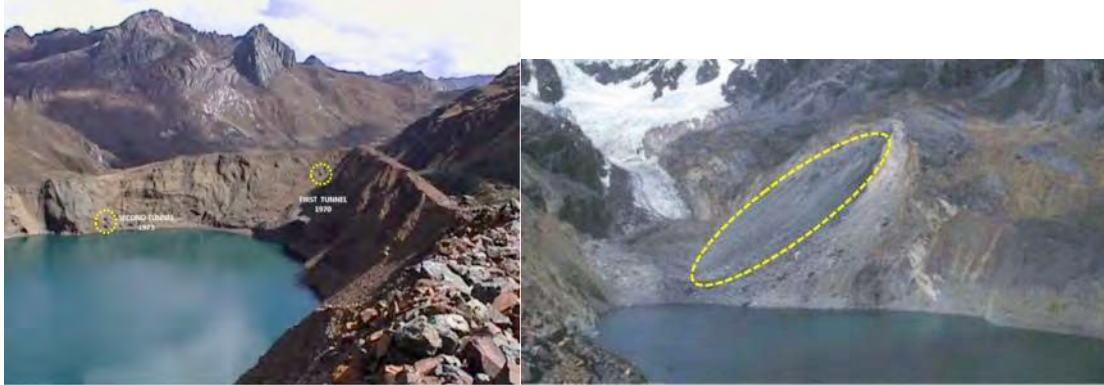
Safuna Alta Lake. Left: Locations of the two tunnels drilled into the moraine in the early 1970s as the lake's level dropped on its own. Right: The source of the landslide in 2002 that launched a wave at least 80 meters in height. Photos: César Portocarrero (1974)
