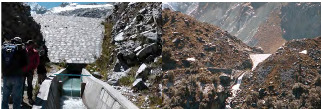
Llaca Lake's safety dam and sluice in 2013. Photos: John Harlin
