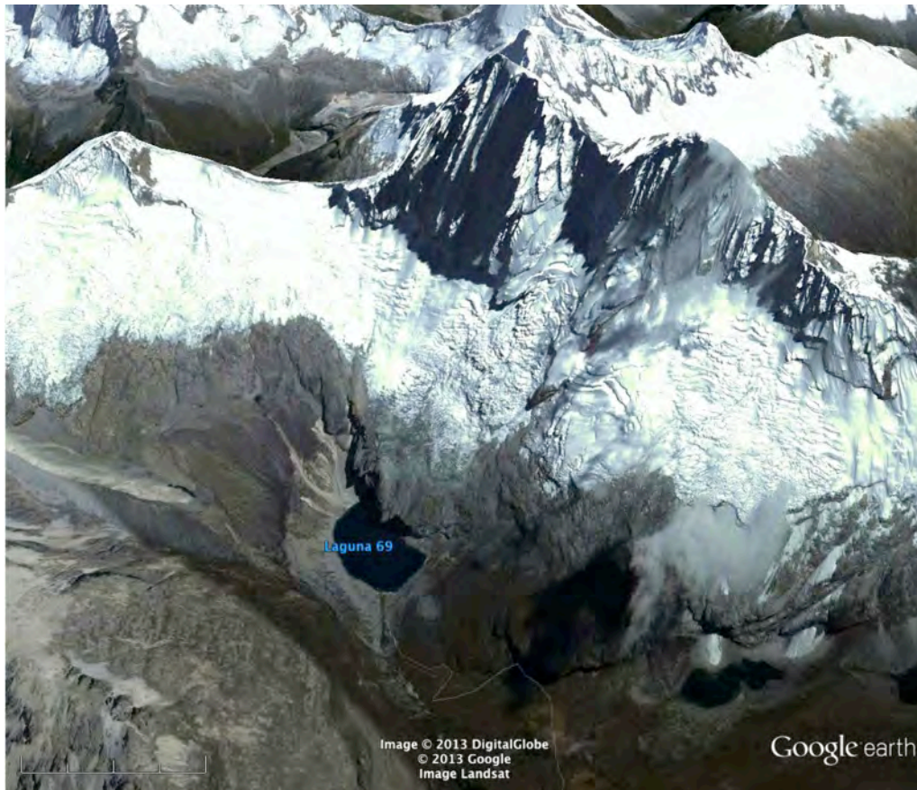
Lake 69 is in the direct fall line from glaciers on Chacaraju Peak (6,112 meters).
