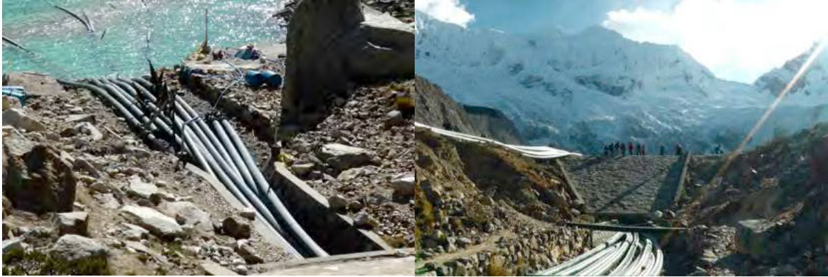
Palcacocha Lake in 2013 showing the siphon pipes entering (left) and exiting the tunnel under the dam. Photos: John Harlin
