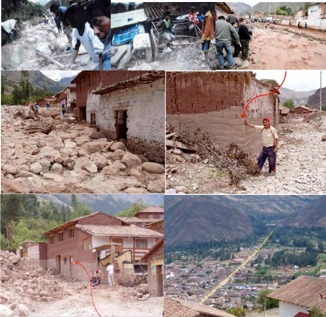
Top row: Photos from the flood of the Chicón River in San Isidro and Urubamba resulting from the Riticocha GLOF on 17 October 2010. Middle row: Debris and flood lines on walls in Urubamba in 2010. Lower right: The path the Chicón River took through Urubamba in 2010. Top row photos: Municipality of Urubamba. Other photos: César Portocarrero
