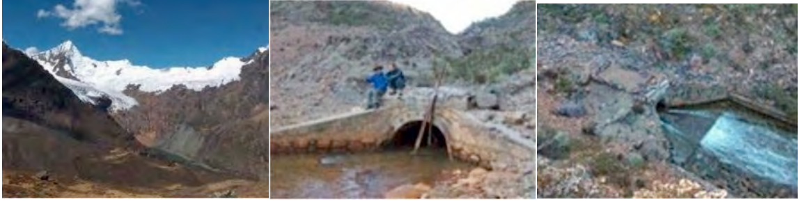
Tullparraju Lake showing its steep flanks and the hanging glacier above. Middle and right photos show the entrance and exit of the drainage tunnel. All photos from 1974: César Portocarrero
