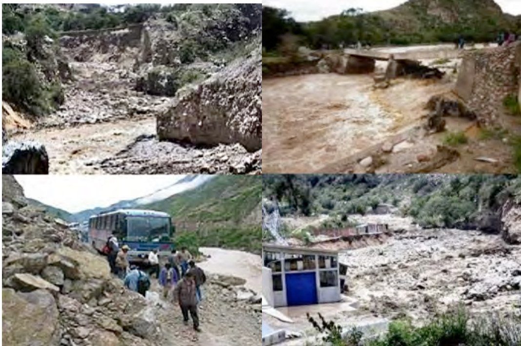
Damage in the Santa Cruz valley downstream from Jatuncocha during the 2012 GLOF. Photos: Hidroeléctrica Santa Cruz
