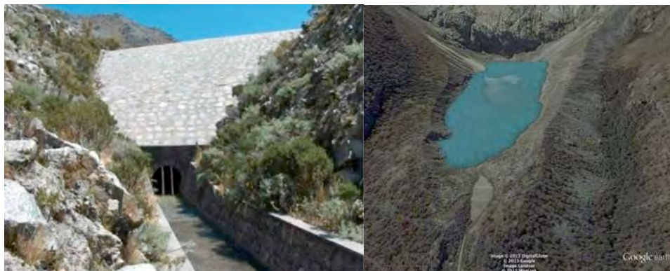
Huallacocha's completed safety dam from below (1978) and above (2013). Photo: César Portocarrero
