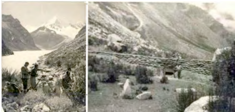
1951 photos of surveyors and a sand bag dam built as a temporary barrier below Lake Parón. Photos: Glaciology Unit Office Archives
