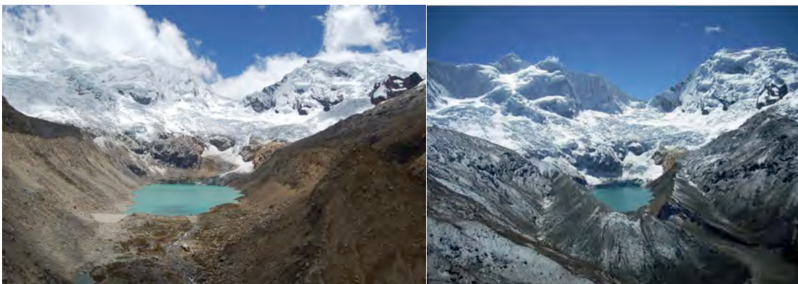
Left: Palcacocha Lake in 2013 taken from the top of the moraine. The two safety dams can be seen. The dam on the right contains the drainage pipes. Photo: César Portocarrero. Right: Palcacocha Lake in 2008 showing its enclosing moraine; the 1941 breach is visible in the lower right. Photo: Colette Simonds
