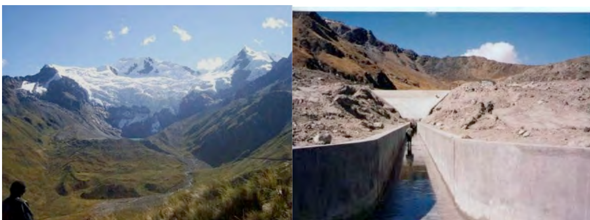
Lazo Huntay Lake showing the still-massive hanging glacier in 1990, and the newly completed safety works in 1990. Photos: César Portocarrero
