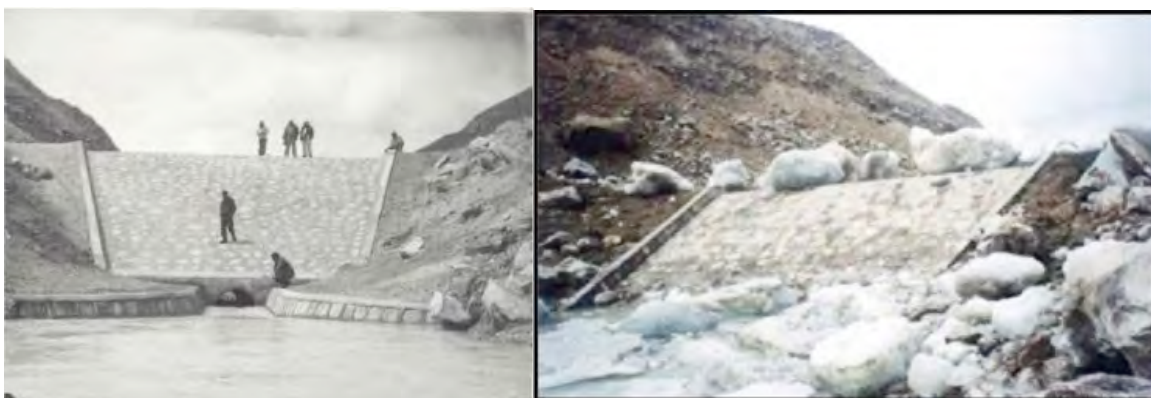
The safety dam on Palcacocha Lake as construction was being completed in 1974 (left) and with ice debris following the 2003 landslide that launched a flood that was mostly contained by the dam. Left photo: César Portocarrero. Right: Glaciology Unit Office Archives
